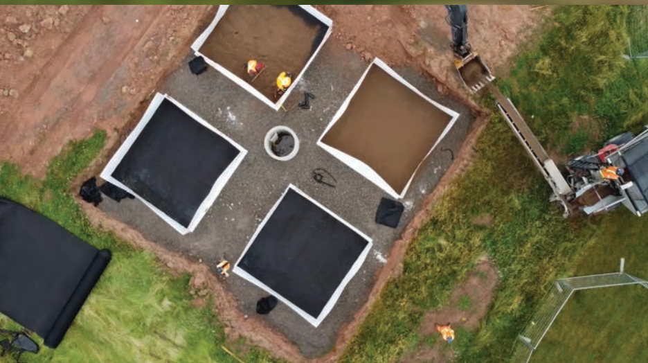
Construction began on Vineland's new TreeCulture Research Park in May 2022.
